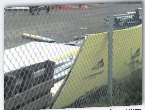
Debris placed against fence - vibration triggered alarm
