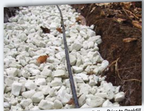
Buried Cable Installation Prior to Backfill
