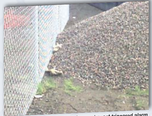
Gravel dumped against fence - impact triggered alarm
